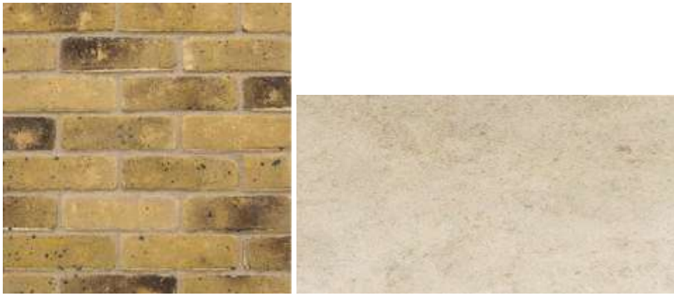
Figure 13: Left – London stock brickwork; middle – lintel/slab facings
