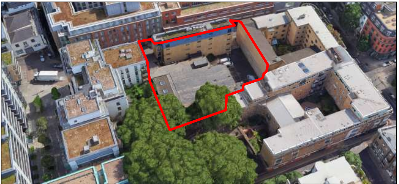
Figure 3: Aerial view of site (in red) from the north looking south
